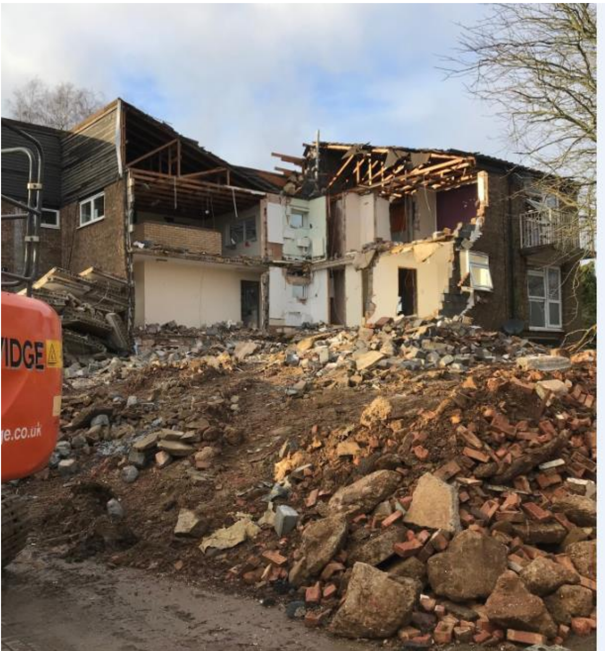
Demolition and site clearance for new homes at Kenilworth (Stirling Close)
